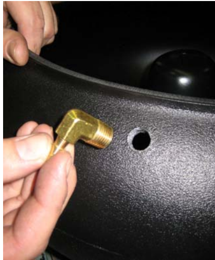
Install 90° inlet fitting to upper hole.
